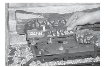
7) Place the notch in Center Log E)02-47 over Log B)02-45 and across the cutout on Log A)02-43.
